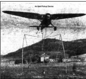
Outbound Marion air mail would be picked up by the mail plane. A cable and hook from the plane would pick up the mail bag as it flew over the station, and mail was delivered by being dropped from the plane with special equipment.
